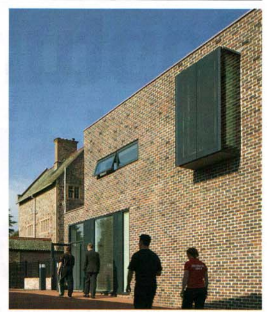
The projecting window on the south elevation showing the perforated aluminium ventilation panel on its main face.
