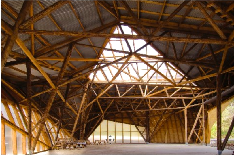
The structure pioneers the use of high-capacity screwed connections within large roundwood trusses.
