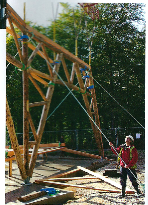
ABOVE: Building full-scale timber structure at Hooke Park.
